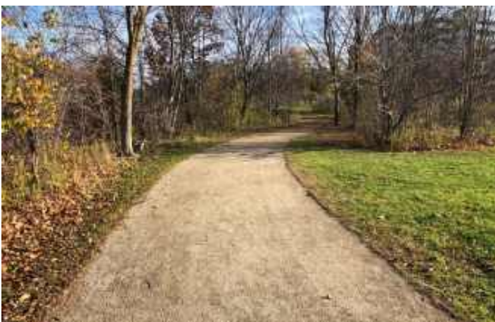
Stabilized aggregate walkways support multiple uses and accommodate the potential for vehicle access.
