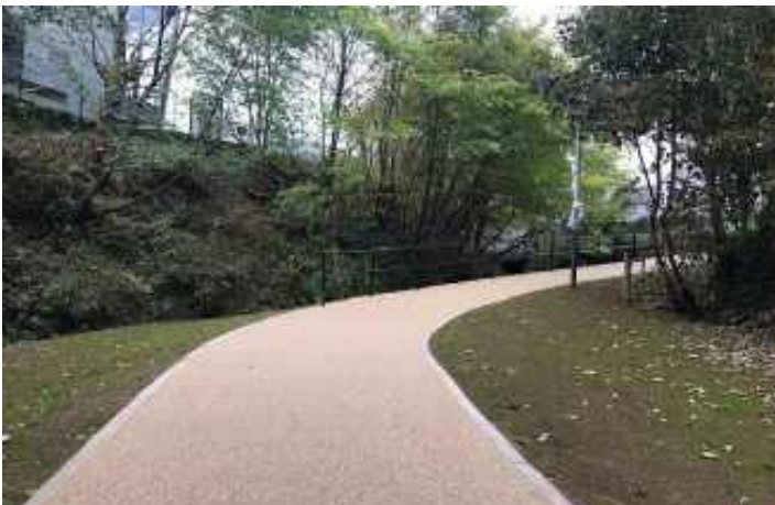
Resin-bound aggregate surfaces provide a firm and stable, permeable surface (ProPave).
