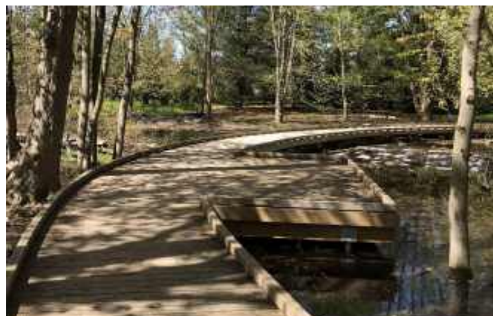
Accessible low boardwalk with observation areas (University of Guelph).
