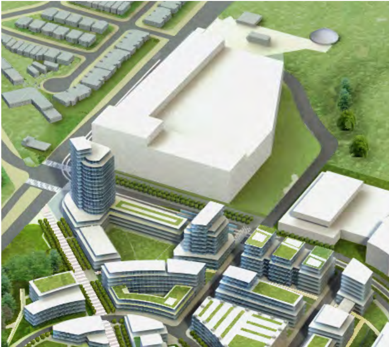
View of the North Campus athletics precinct at the intersection of Military Trail and Morningside Avenue
